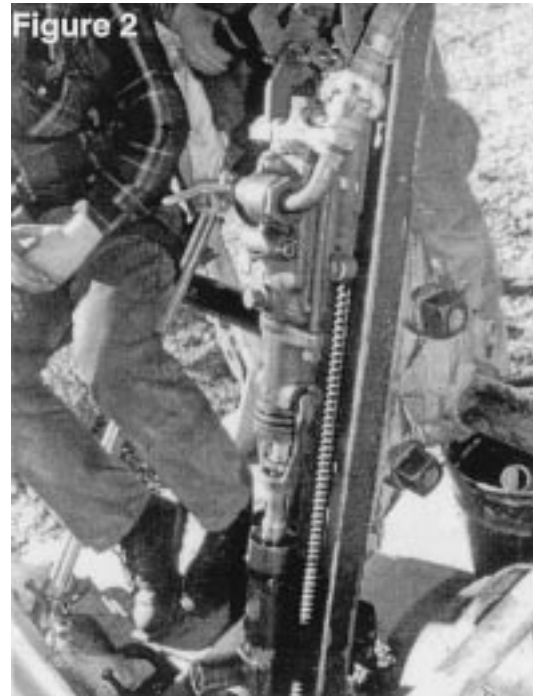
Fig. 2. Pneumatic rock-drill mounted on a pneumatic screw-drive guide system. The screw, which is seen behind the rock-drill, may be turned pneumatically in either direction, driving the rock-drill downward as drilling or pipe-driving proceeds, or upward to back the rock-drill off. The pipe driver is attached to the rock-drill in this photo, and is being used to drive the drill casing into the ground.
